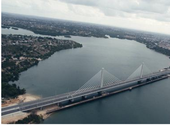
Figure 2.3 View of Kigamboni Bridge Source; Consultant, May 2022
